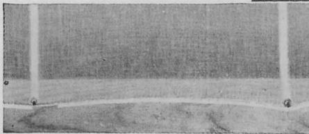
Note how side wall Cloth is attached to baseboard. It is not necessary to use the usual wood strip, thus eliminating dampness and rot.
